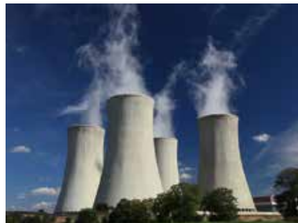
Figure 4 - Cooling tower in the shape of hyperboloid. Source: Science and Entertainment. Available on <http://parquedaciencia.blogspot.com.br/2013/04/conicas-no-coes-intuitivas-e-aplicacoes.html>. Accessed on January 19, 2017.
